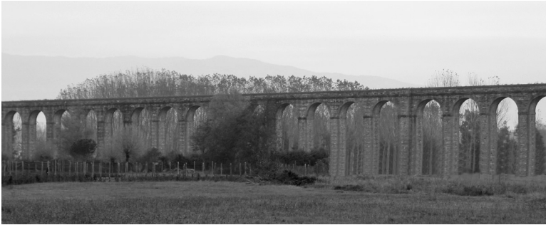
Acquedotto. The aqueduct, designed by Lorenzo Nottolini, was built between 1823 and 1832, and carried water to the city of Lucca. Shown are 18 of its 459 arches.
